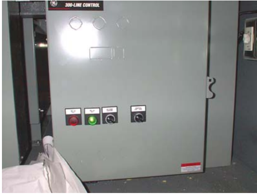
Figure 25: 480V and 120/208V AC Electrical Panels
