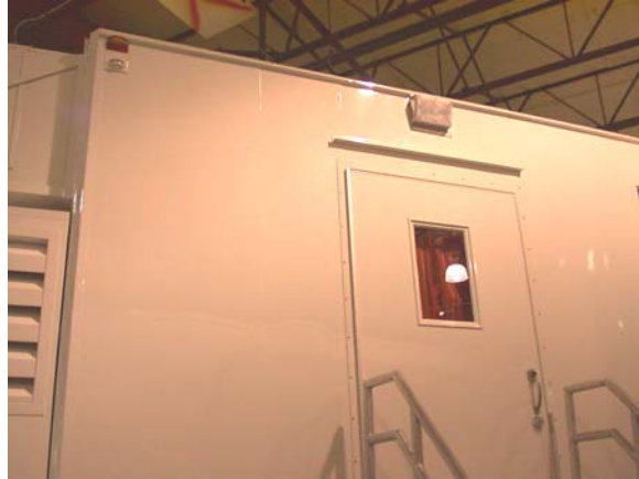
Figure 38: Entry Door Lighting
