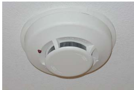
Figure 20: Smoke Detector
