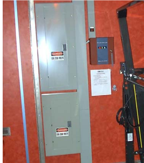
Figure 25: 480V and 120/208V AC Electrical Panels
