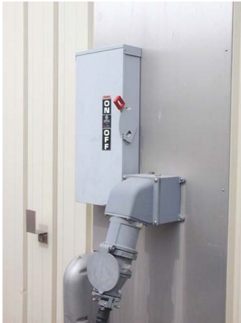
Figure 27: Shore Power Connection
