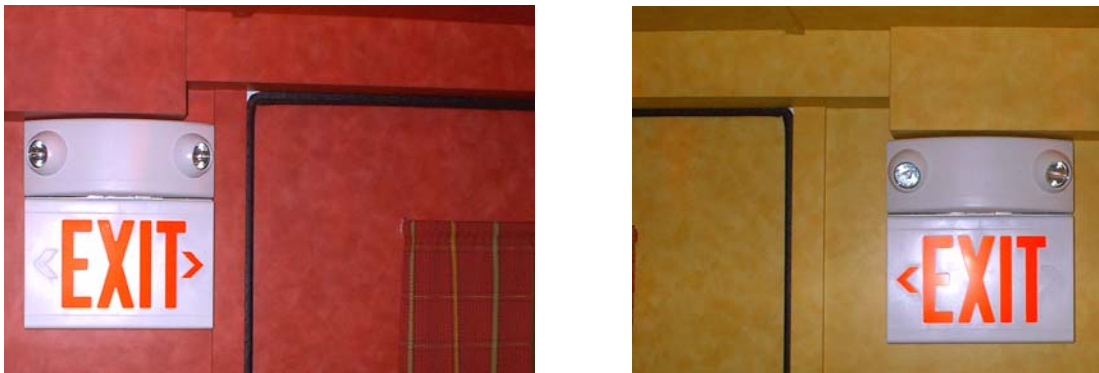
Figure 18: Emergency Lighting
