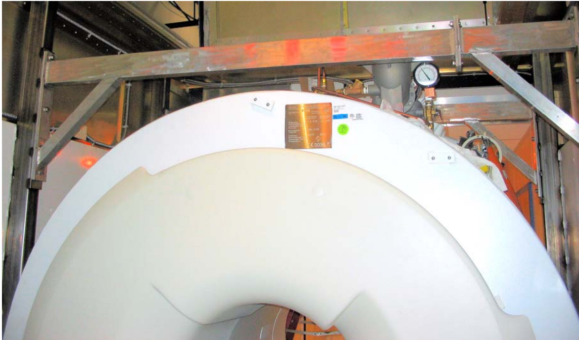
Figure 74:-Cross Brace Assembly Mounted & Secured
