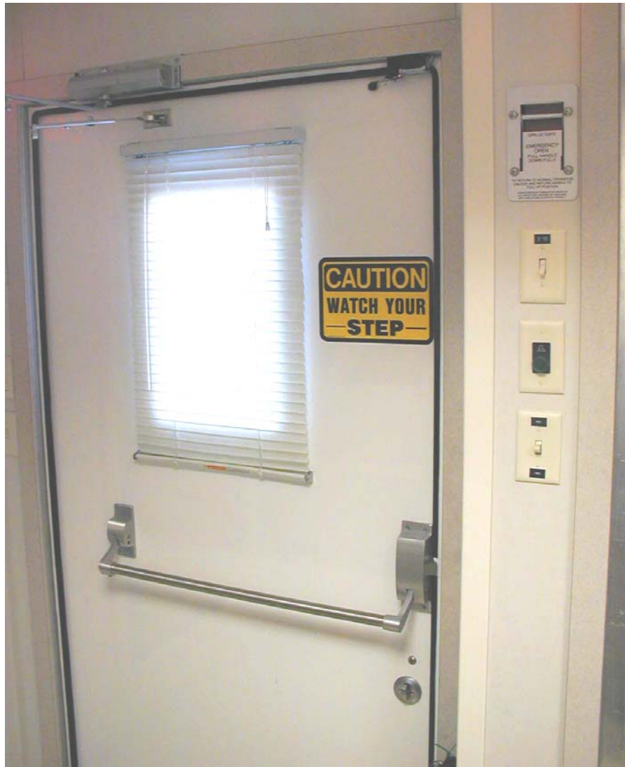
Figure 9: Exterior Staff Door
