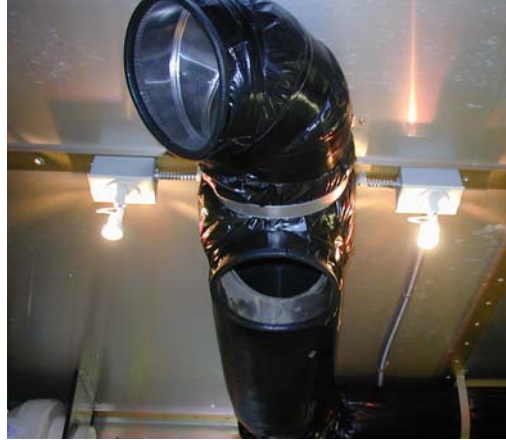
Magnet Room Lighting
