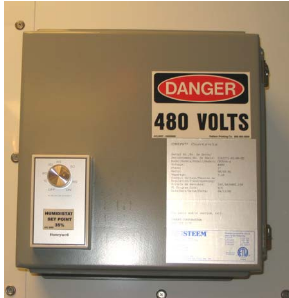
Figure 29: Humidity Controller
