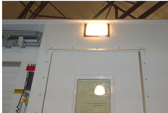
Figure 46: Staff Door Lighting
