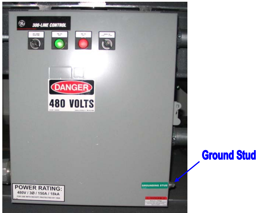
Figure 27: Ground Connection
