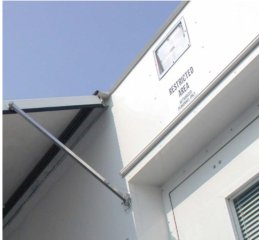
Figure 61: Staff Door Lighting
