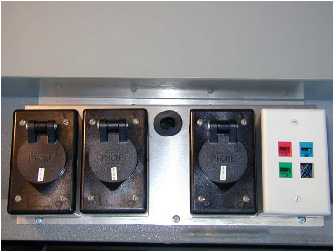
Figure 25: Phone and Data Line Connections (Typical)
