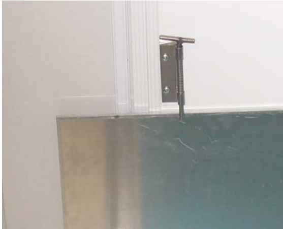
Figure 43: Inner and Outer Patient Door Floor Transition Plates Up and Locked
